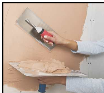
PLASTER over Plaster-Grip Primer.
